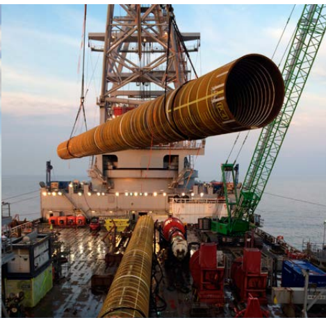
Monopile foundation of a met mast.
