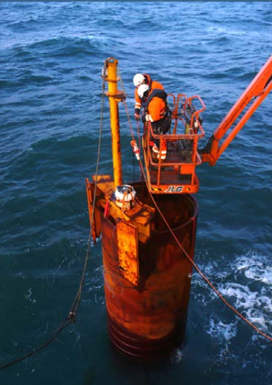
Safe-keeping of the cable connectors of an instrumented foundation for later continuation of the measurements.
