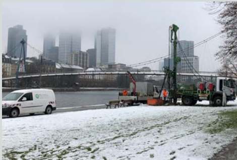
Subsoil investigations on the banks of the river Main in Frankfurt.
