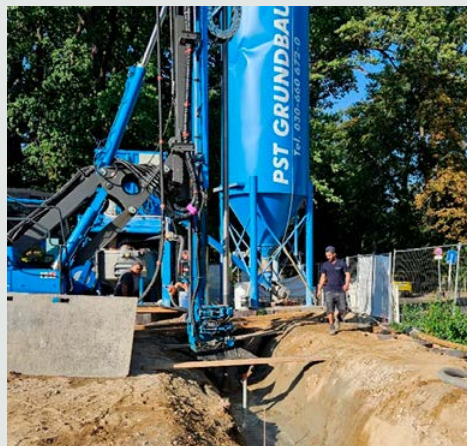
Jet grouting on the construction site in Regattastrasse.
