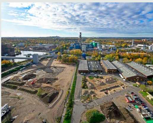
The Reuter power plant in Berlin is being extensively upgraded.
