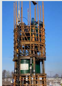
GRL-Cell installation within the steel reinforcement and cable management
