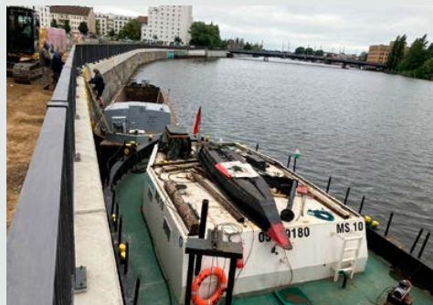
Renovation work on the riverbank wall.
