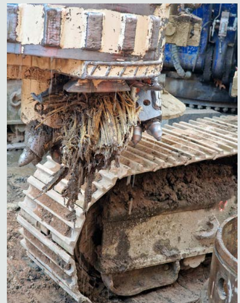
Old wooden piles complicated the drilling work.
