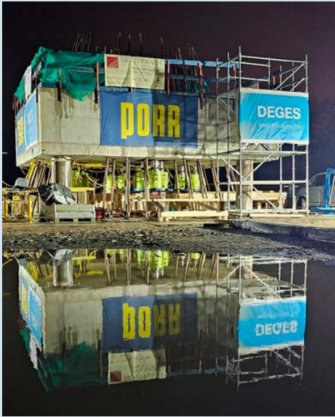
Test load for the new A26 motorway.
